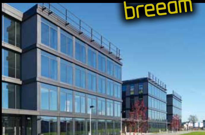
Enterprise Park, Kraków
